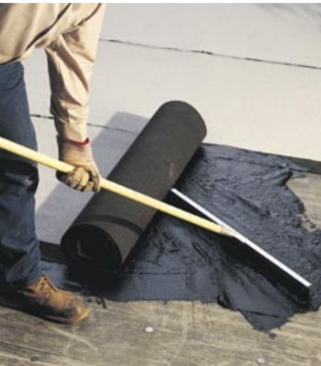
TAM-PRO Premium SBS Adhesive squeegee applied. TAM-PRO M3 Adhesive spray or squeegee applied.
